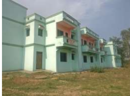
Main Building block
