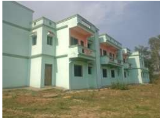
Main Building block
